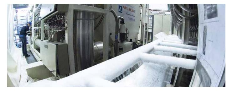
The cooling and operation of superconducting RF cavities and magnet systems for particle accelerators and magnets for detectors requires large quantities of cryogenic fluids. (CERN-EX-0606020-01)
